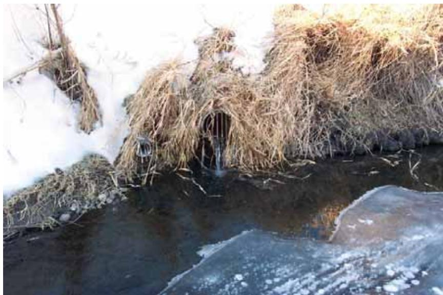
**Figure 8 – Outlet of a straight pipe from a community in southeast Minnesota.**
